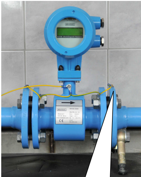
Metal pipeline Grounded to flanges
