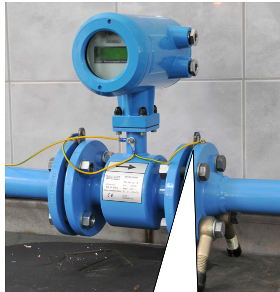
Plastic pipeline Grounded to grounding rings
